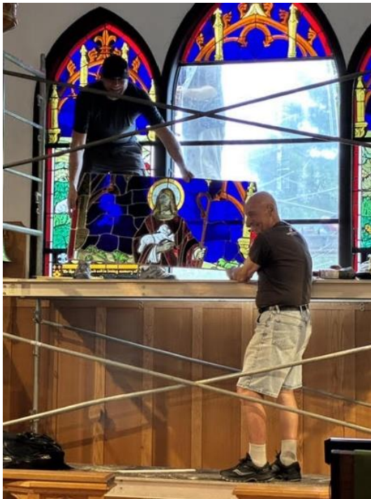
Warden Art MacDonald helping to install the window
